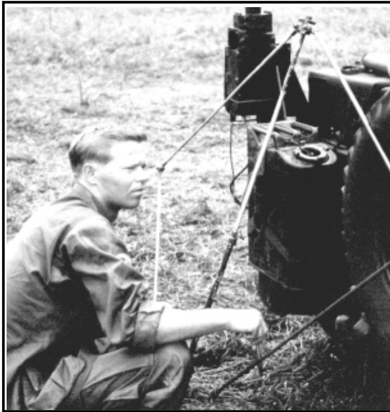
Orville (Butch) Browning putting together the diamond shaped antenna for our direction finding radio. The antenna was rotated as we listened in headphones for the direction of the enemy signal.
